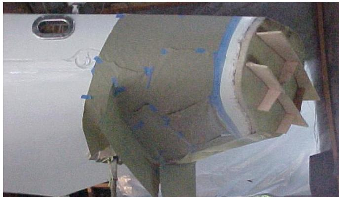
Once Skip had finished spraying the Fleet White Awlgrip on the port side, it was time to work with the transom again. Here, he has taped off the hull to protect the new finish. He coated the transom in wax and then laid up two layers of fiberglass. He formed wood to it to help make it stiff. Once it set, he was able to remove it and lay it on his workbench. This time he waxed the inside of the mold and was able to lay up several layers of
