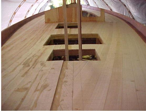
On May 30<sup>th</sup>, I took this picture showing the first layer of cedar in line with the sheer and half of the second layer laid parallel to the centerline. The first layer, Skip fitted dry and glued it to the beams. The second layer he glued over the whole deck, without the tongue and groove. He will finish-up the second layer within the a few days and then begin a different third layer.
