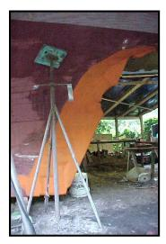
Once again, understanding all the thicknesses of future work Skip cut away about 4 inches of wood off the back of the boat. He then painted it with Red Lead in preparation for the fiberglass.
