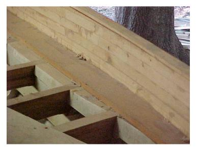
The first strip went down on the deck, clamped tight to the temporary molds, then fastened to the deck. Each layer he then built upon the one before as he fastened it all with glue and 3 & 1/2" nails, every 6 inches.
